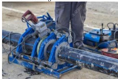
Gambar 4 But Fusion Welding
