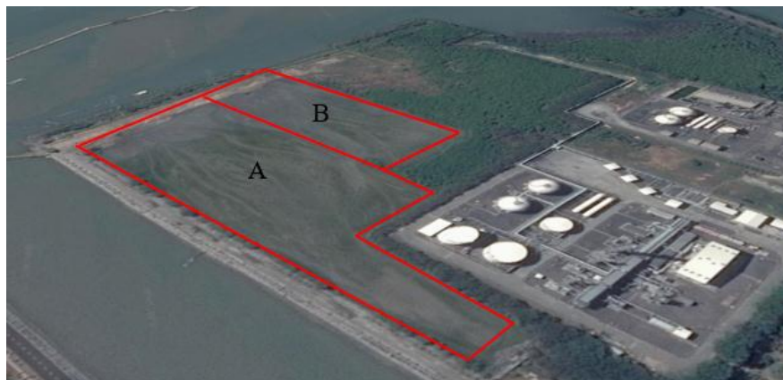
Gambar 1. Lokasi Storage Pond Lumpur Intake
